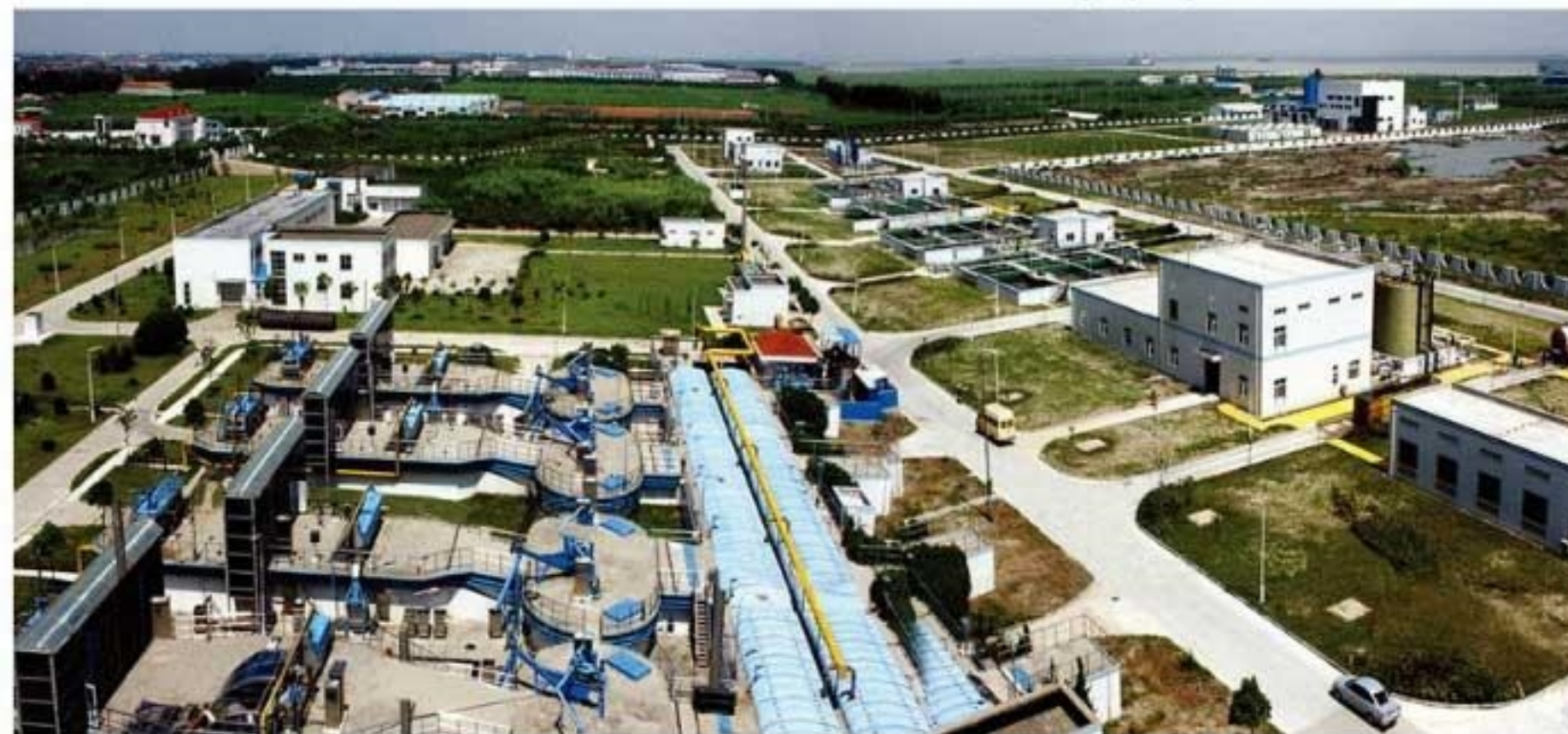
白龙港污水厂 Bai Long Gang Sewage Water Treatment Plant
